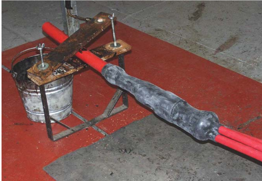
3 CORE POLYMERIC TO 3 SINGLE CORE TRIFURCATING JOINT
